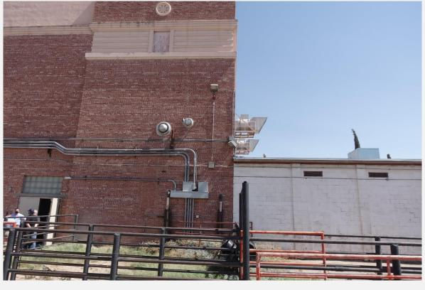
Low canopy at south end of Coliseum restricts truck access/movement. Suggest replacing canopy with new loading area and back-of-house support space.
