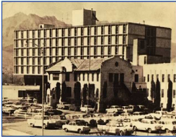
Construction completed on 300-bed R.E. Thomason General Hospital
