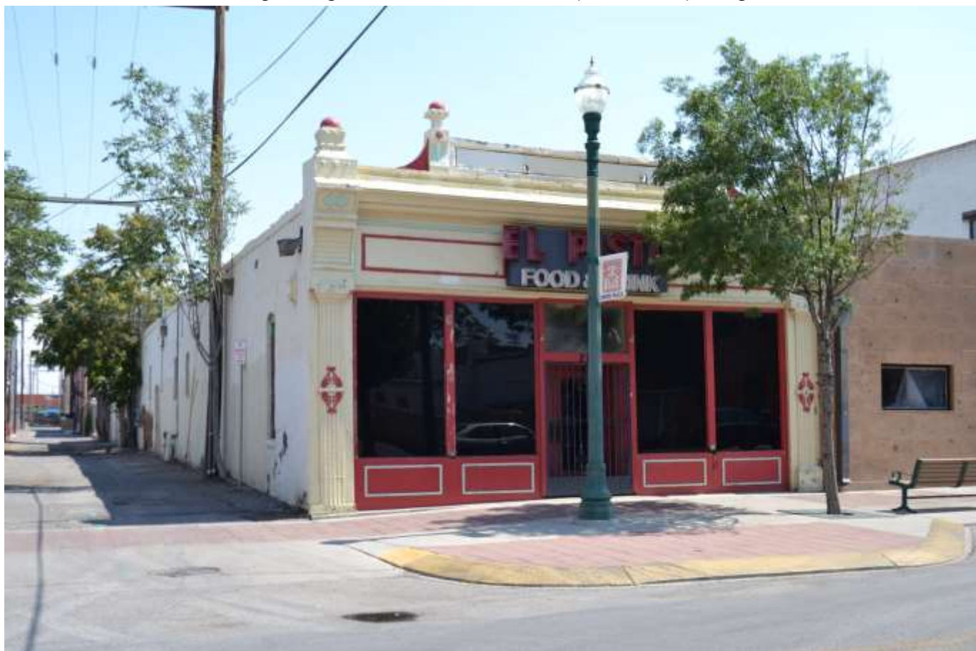
Photo no. 54. View of contributing building at 212 West Overland Avenue (Resource 156), facing south.
