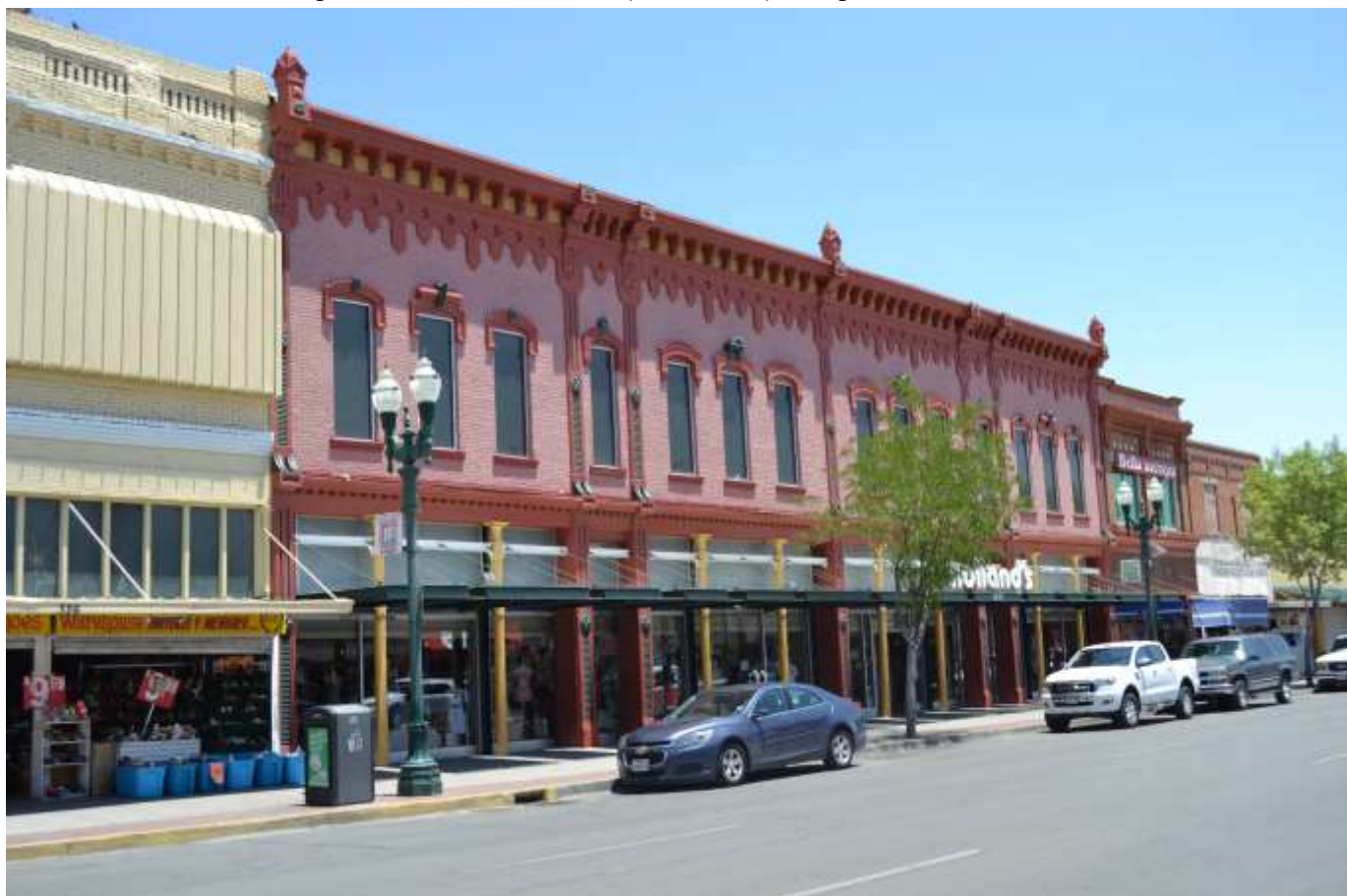
Photo no. 31. View of building at 402 South El Paso Street (Resource 47), facing southeast.
