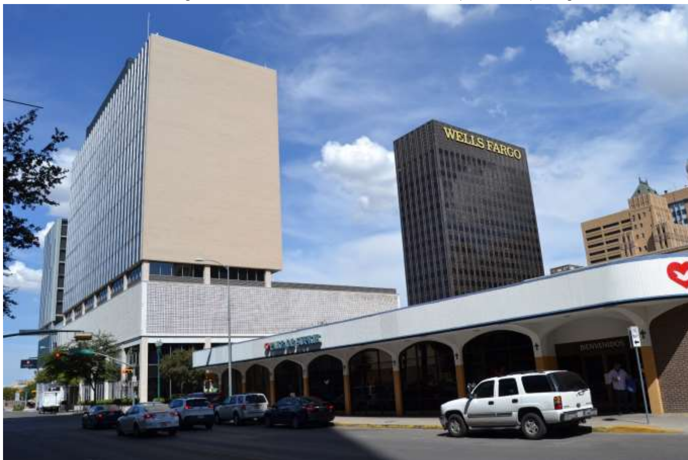
Photo no. 69. View of contributing Downtowner Motor inn at 300 East Main Street (Resource 78), facing north.
