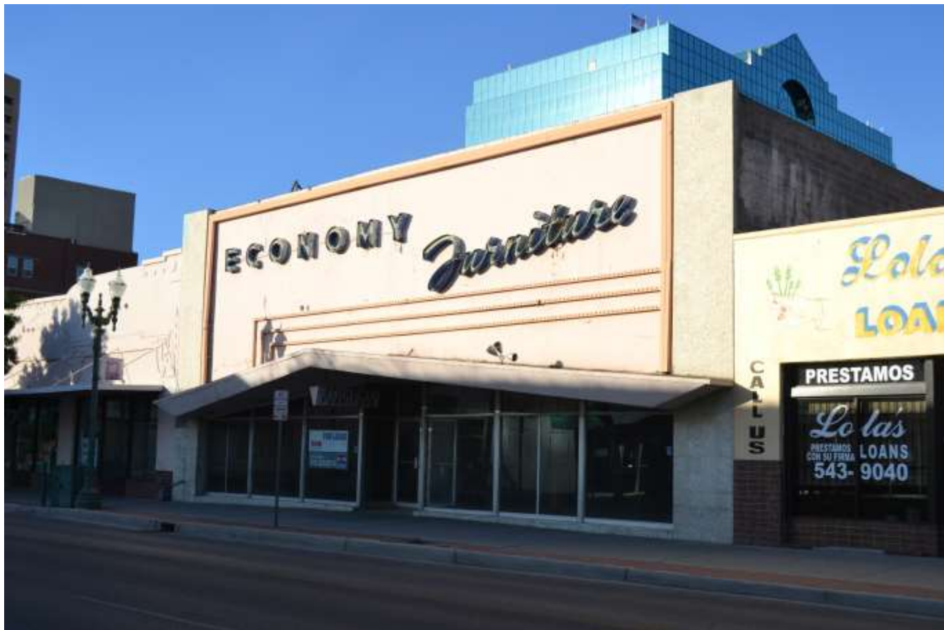
Photo no. 60. View of contributing Economy Furniture building at 210 South Stanton Street (Resource 242), facing northeast.
