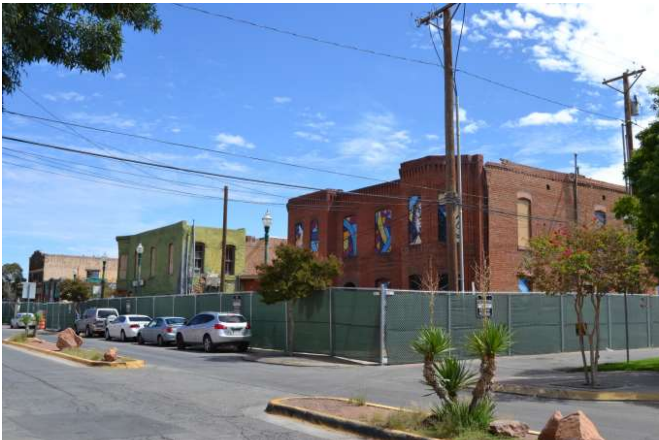
Photo no. 48. Contextual view of West Overland Avenue in Duranguito currently fenced, facing southeast.
