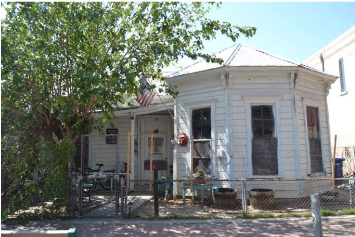
Photo no. 30. View of wood-frame house at 400 West Overland Avenue (Resource 167), facing south.
