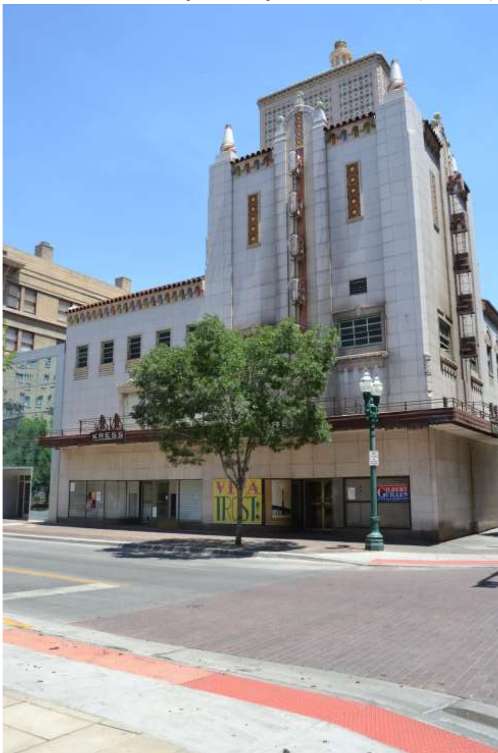
Photo no. 57. View of contributing Kress Building at 211 North Mesa Street (Resource 85), facing southeast.
