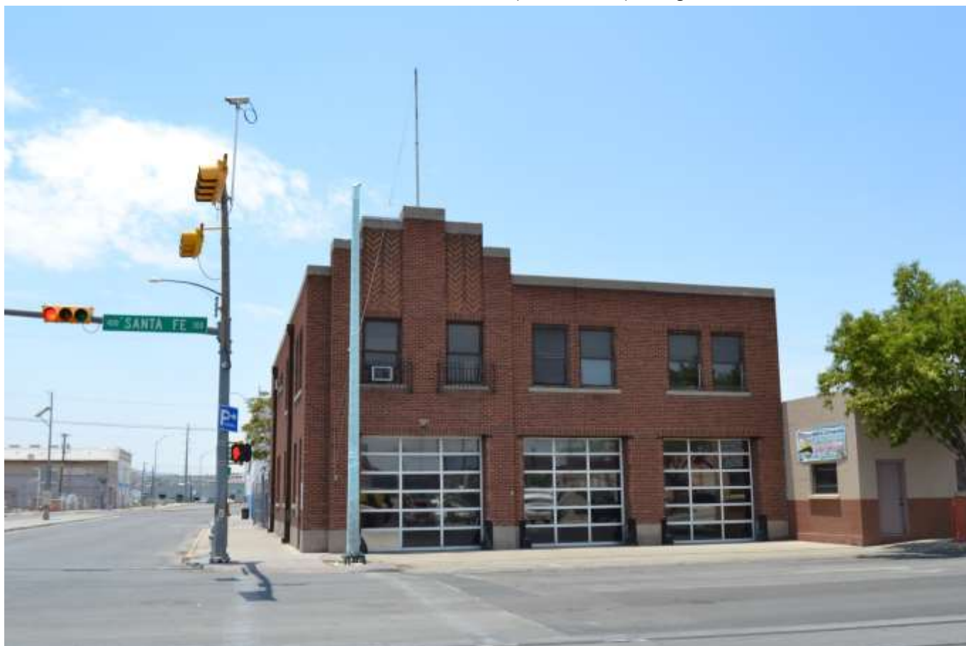
Photo no. 22. View of the fire station at 331 South Santa Fe Street (Resource 223), facing west.
