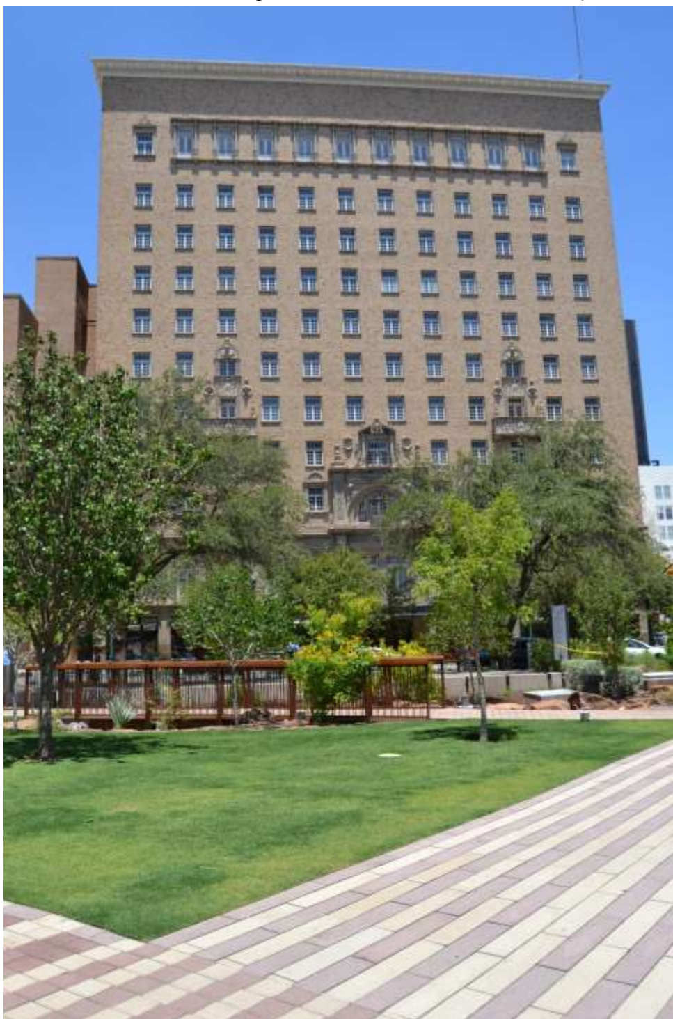
Photo no. 66. View of contributing Hotel Orndorff at 310 North Mesa Street (Resource 87), facing northeast.
