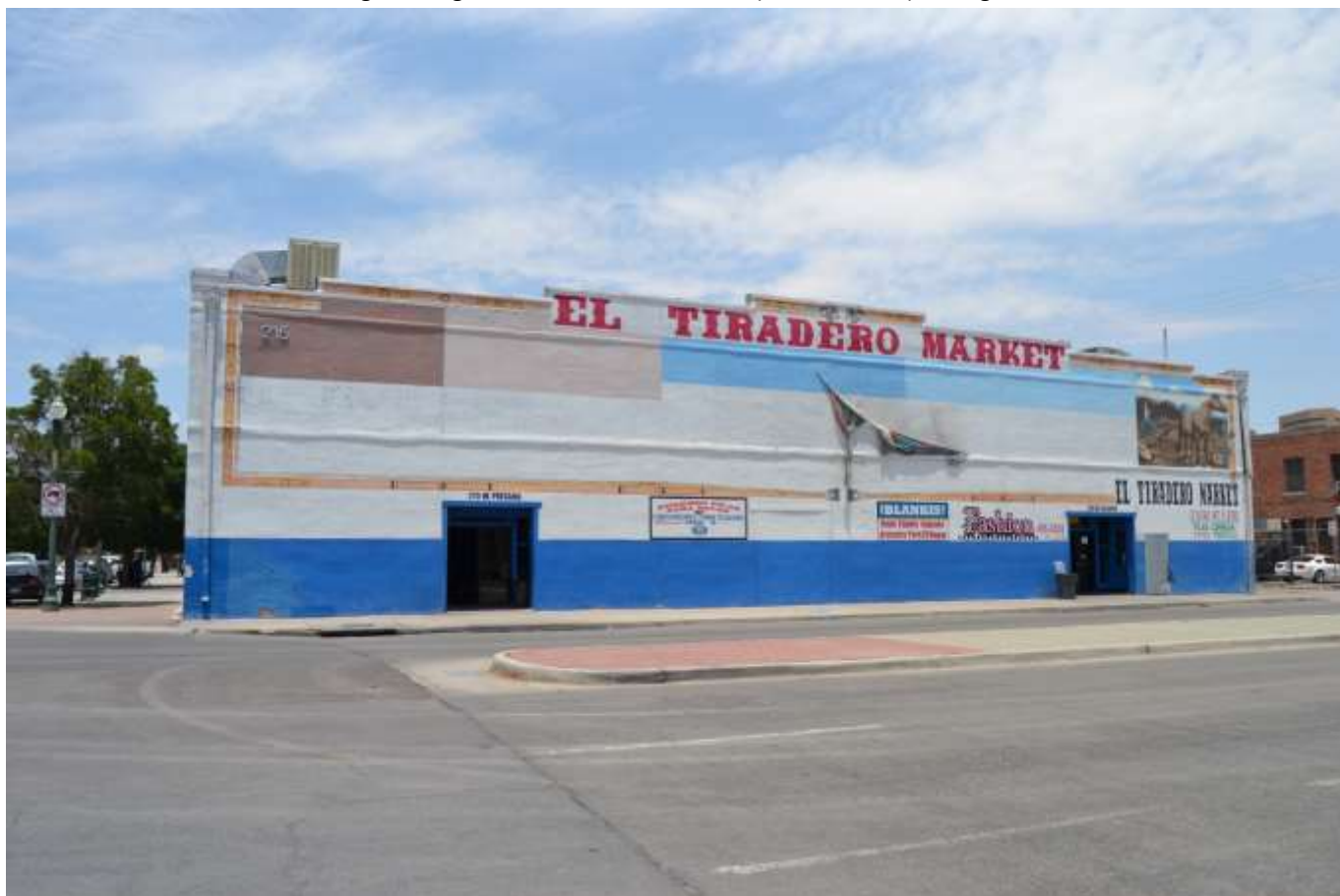
Photo no. 58. View of contributing building at 215 West Paisano Drive (Resource 178), facing north.
