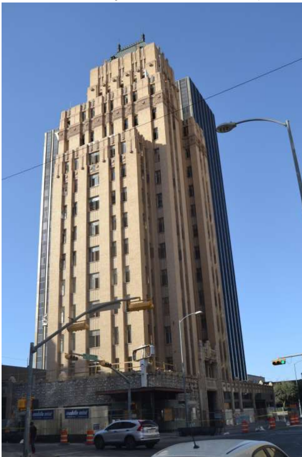
Photo no. 68. View of contributing O.T. Bassett Tower at 301 Texas Avenue (Resource 262), facing north.
