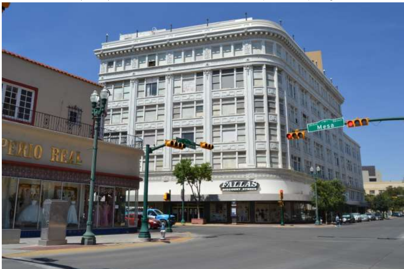
Photo no. 42. View of Popular Department Store at 301 East San Antonio Avenue (Resource 193), facing northeast.
