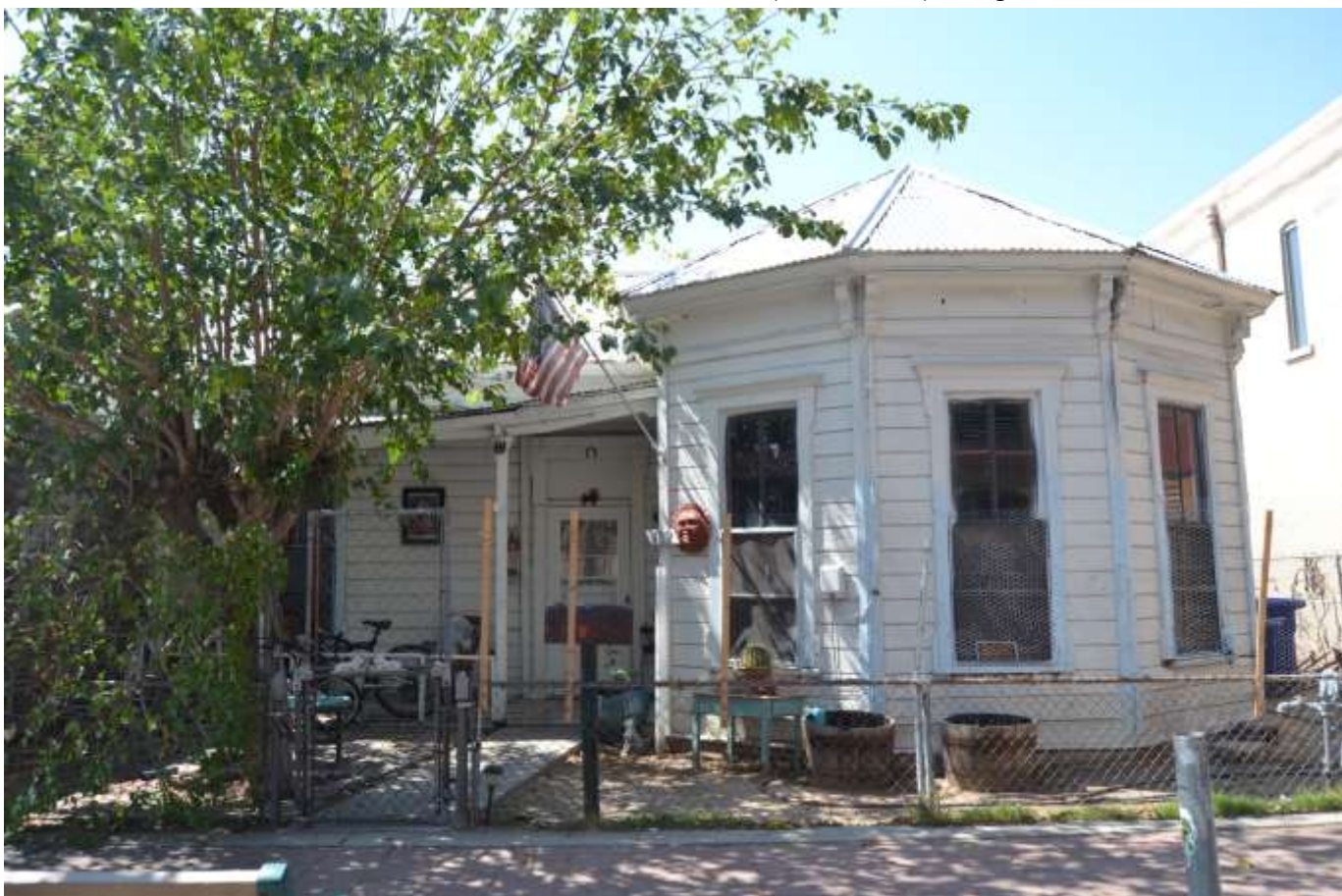
Photo no. 30. View of wood-frame house at 400 West Overland Avenue (Resource 167), facing south.
