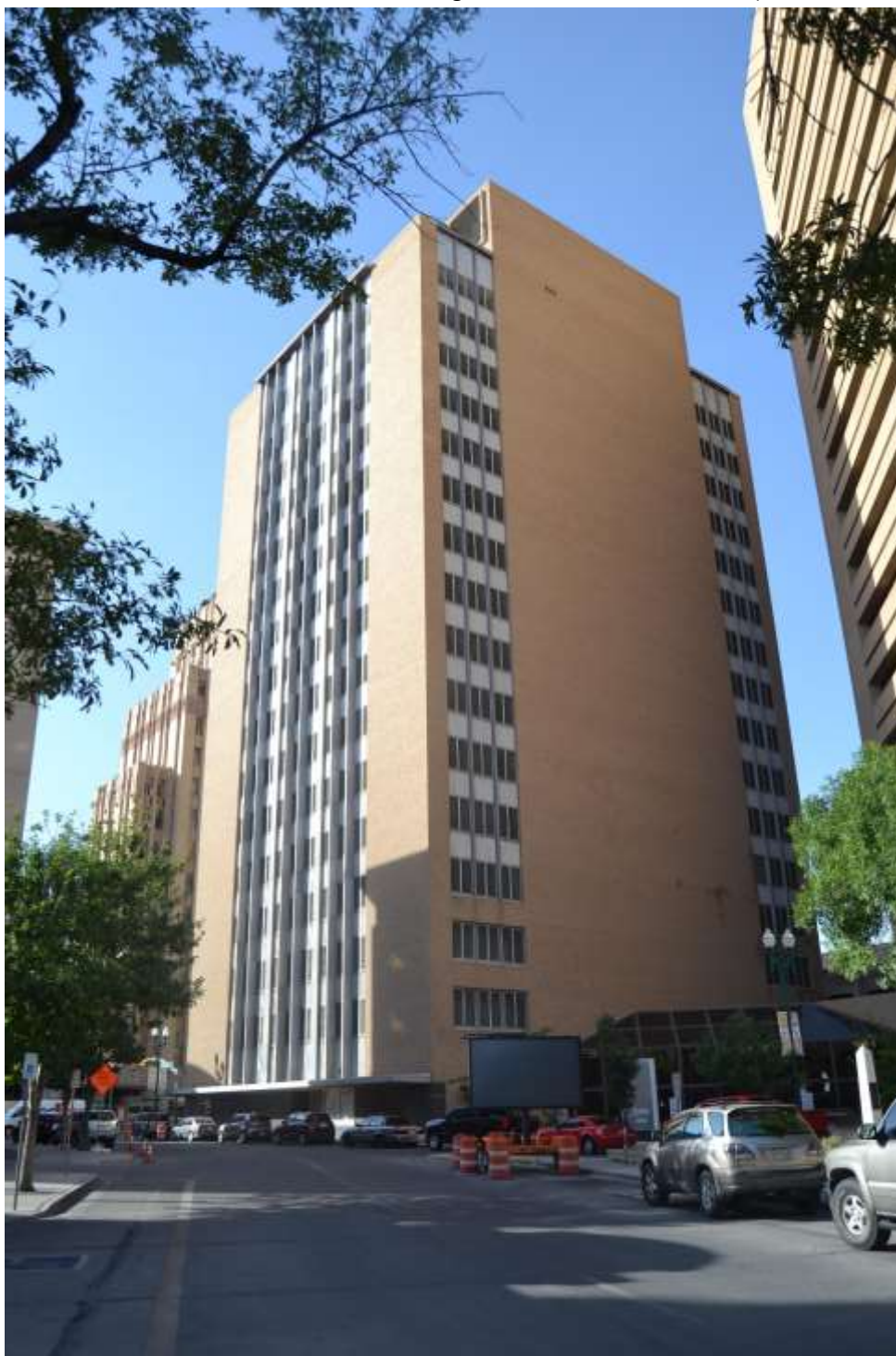
Photo no. 46. View of the Blue Flame building at 120 North Stanton Street (Resource 226), facing north.
