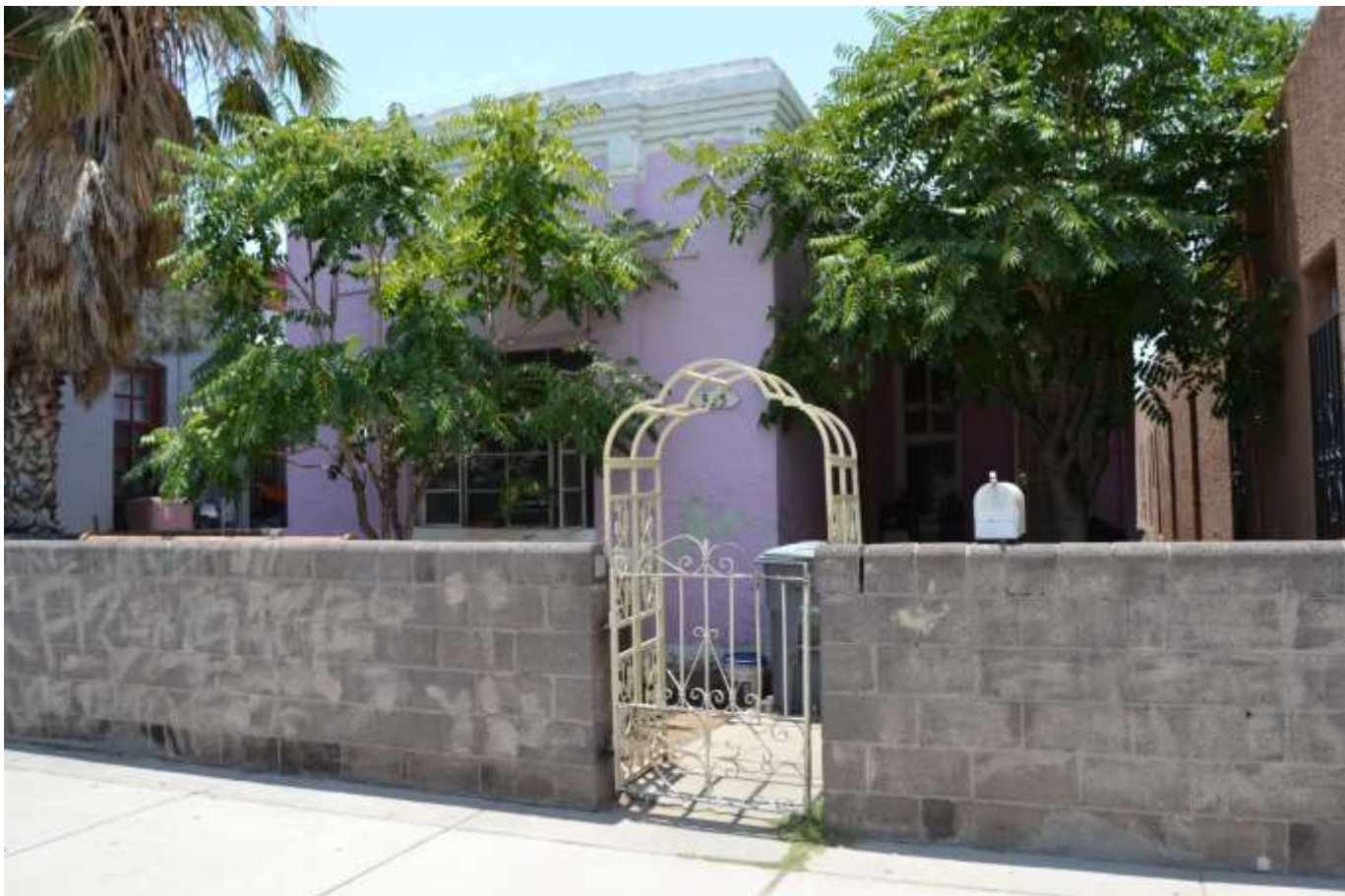
Photo no. 36. View of residence at 325 Chihuahua Street (Resource 12), facing west.
