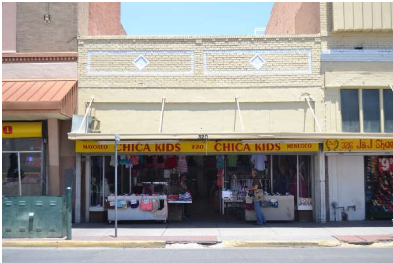
Photo no. 63. View of contributing building at 320 South El Paso Street (Resource 44), facing east.
