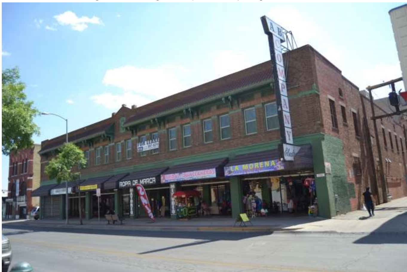
Photo no. 13. View of building at 215 South Oregon Street (Resource 131), facing southwest.
