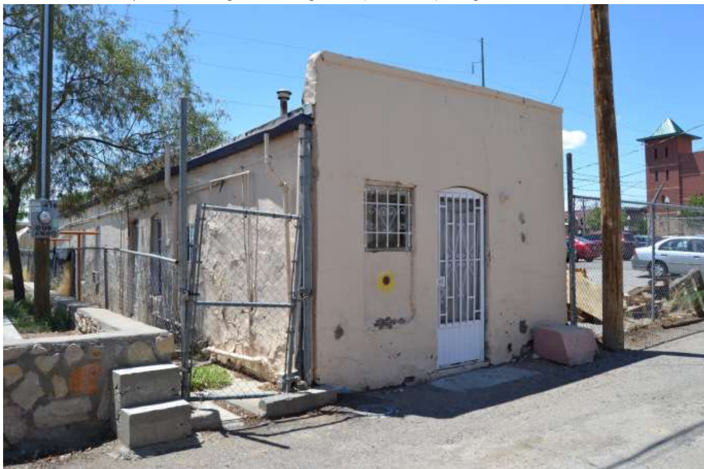
Photo no. 20. View of apartment building at 414 Durango Street (Resource 20), facing northwest.
