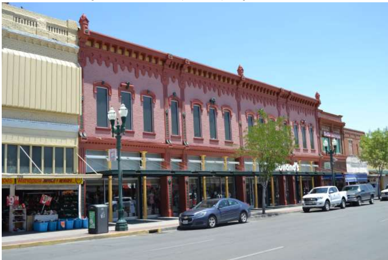
Photo no. 31. View of building at 402 South El Paso Street (Resource 47), facing southeast.
