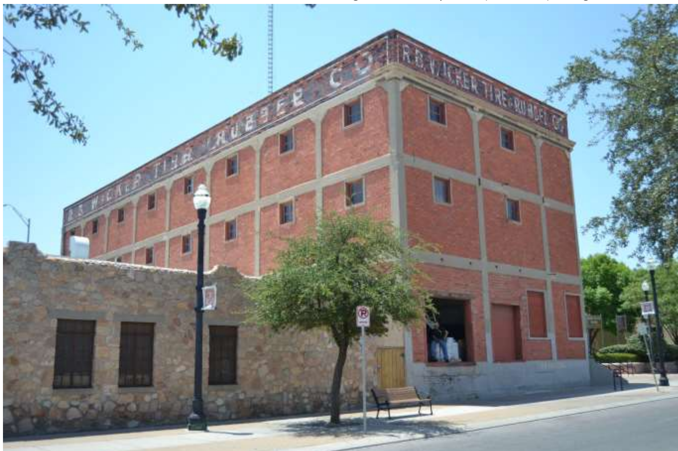
Photo no. 21. View of the R.B. Wicker Tire and Rubber Co. building at 201 Anthony Street (Resource 3), facing northwest.
