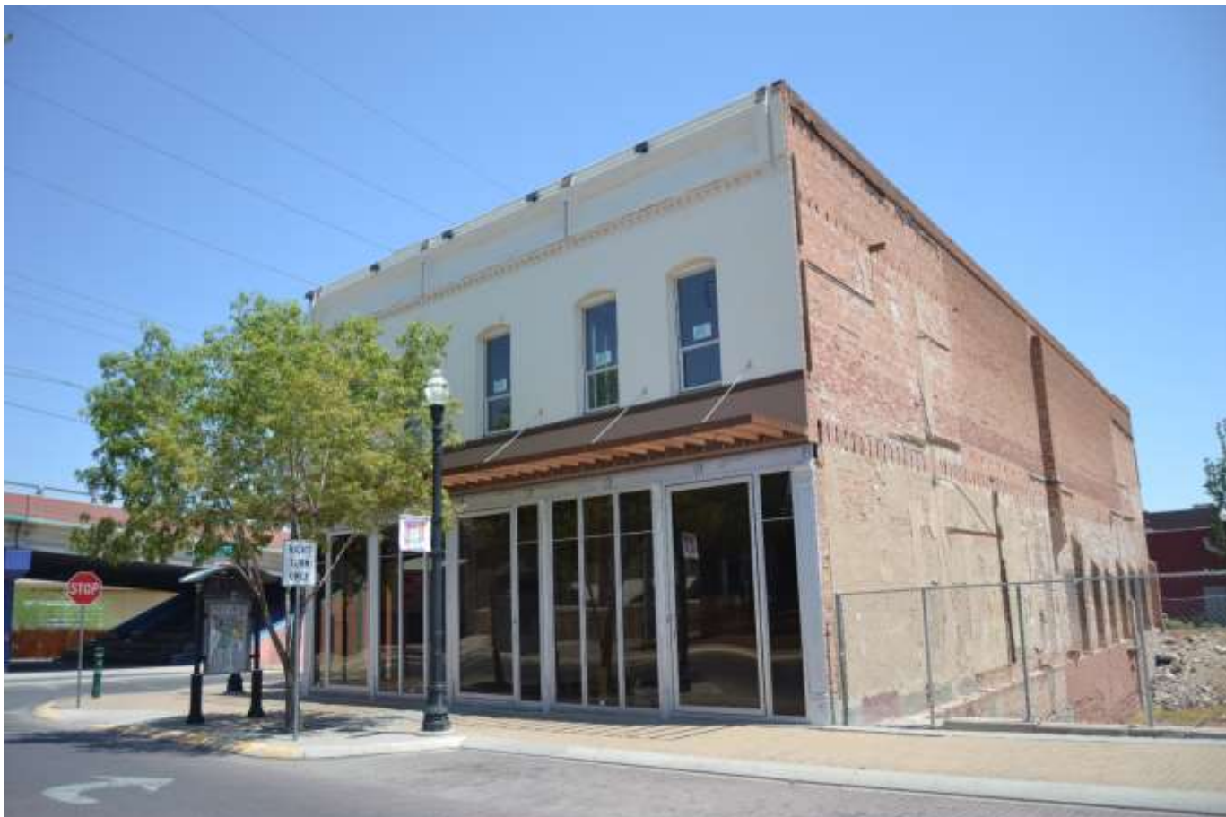
Photo no. 62. View of contributing building at 500 West San Francisco Street (Resource 213), facing southeast.
