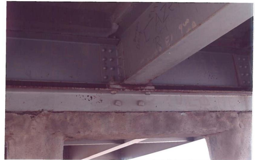
Structural Detail Showing Minor Corrosion of Beam
